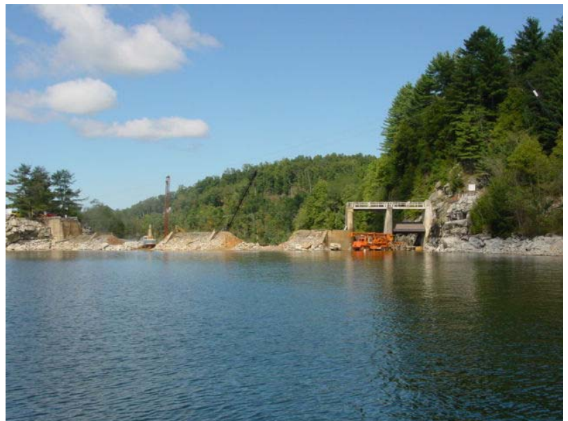
Above: In a photograph taken September 2nd 2002 by Keith Dixon while out fishing, most of the road over the dam is clearly gone, along with some of the dam itself. Please see page 5 for a more recent picture from the Crossroads Chronicle.
