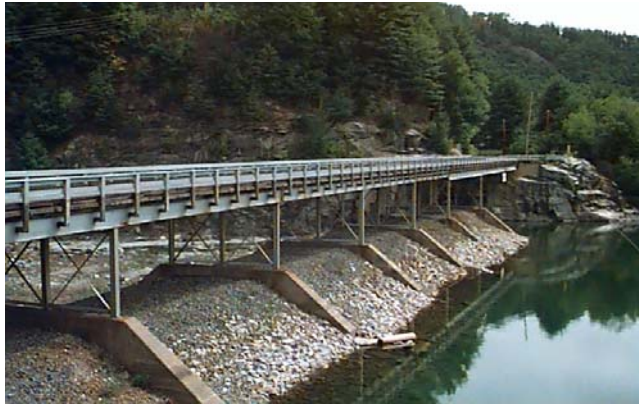
Good news: The bridge reconstruction won't be started until Sept. 2001
